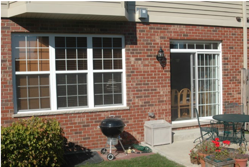
Back yard with 10' x 10' concrete patio
